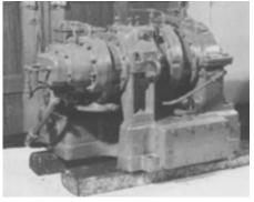
**1943** The first screw compressors are being built
